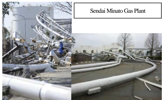
Figure 8 Severe damage at Minato Gas Plant
